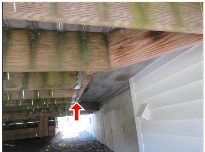
Ledger board attached to house overhang
